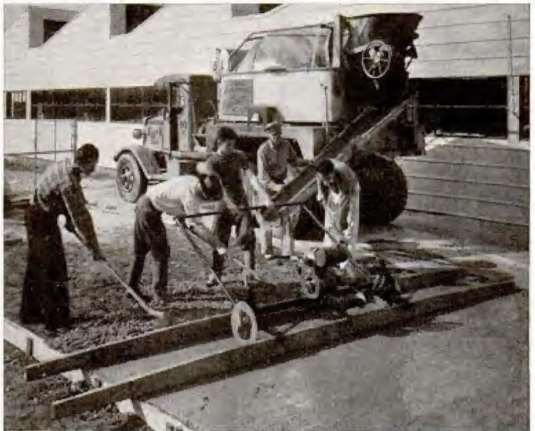
Motorized unit shakes concrete, bringing water to the top for drying
